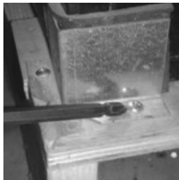
Image 1 Removing bracket from skid
